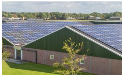
▲ Roof-mounted solar panels
