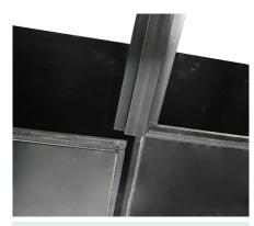
A connection profile is used to simply click the wall ends together.
